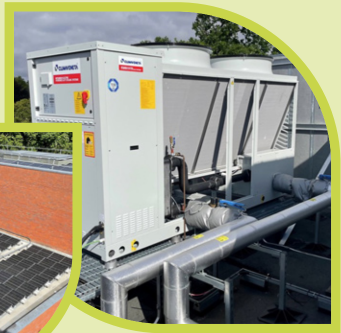
RIGHT: AIR SOURCE HEAT PUMPS INSTALLED AT CAMPUS WEST
