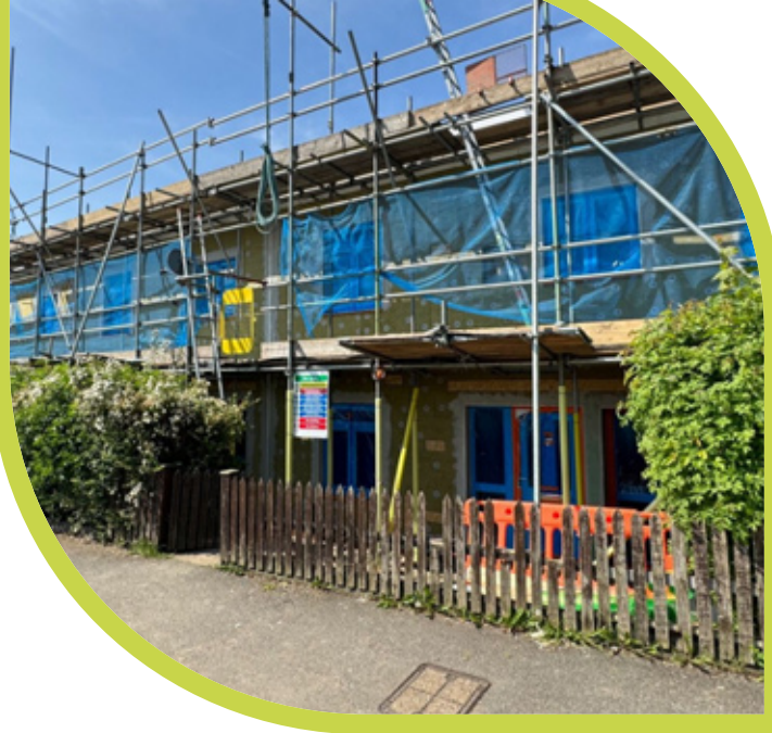
ABOVE: RETROFIT WORK AS PART OF THE SOCIAL HOUSING DECARBONISATION FUND
