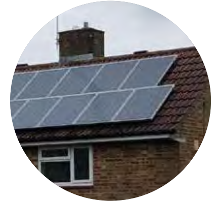
SOLAR PANELS, ALTHOUGH THEY SHOULD BE LESS INTRUSIVE THAN HERE
