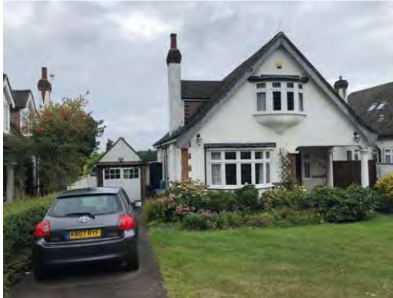
Figure 84: On-plot side parking in Northaw.
