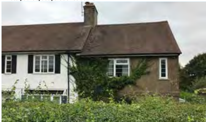
White painted and brick finishing facades.
