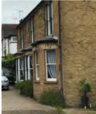
Ground Floor Bow Windows in Northaw.
