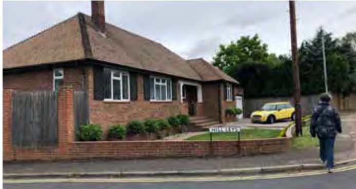
Modern low brick walls dividing private front gardens from the pavements
