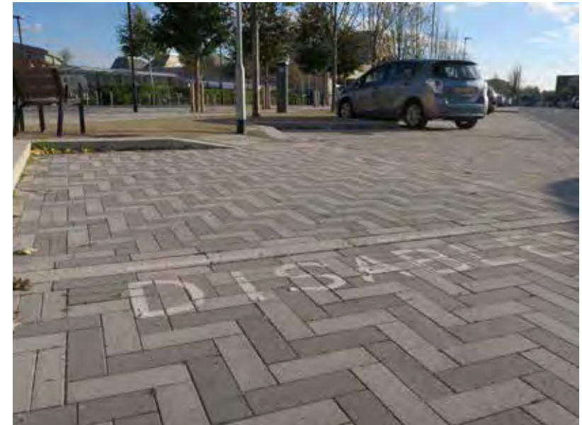
Figure 87: Disabled parking bay with ramp for easy wheelchair access.
