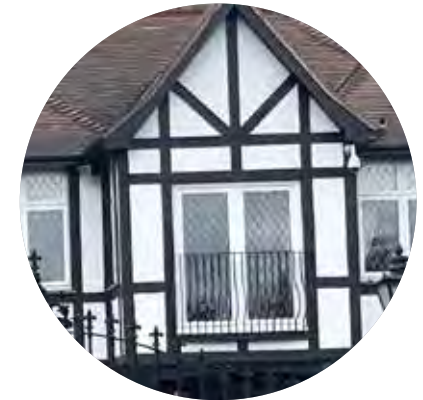
TIMBER FRAMING AECOM
