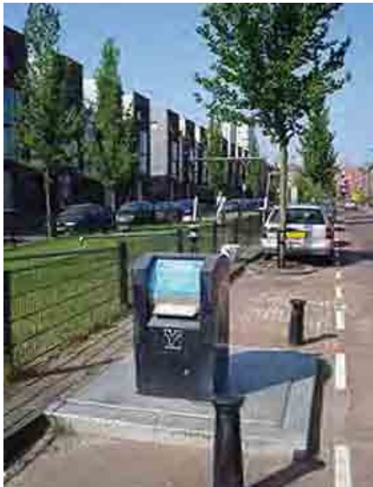
Figure 6.21 Refuse disposal point discharging into underground collection facility.
