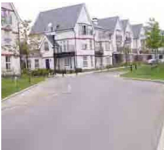
Figure 9.3 Street with no centre lining.
