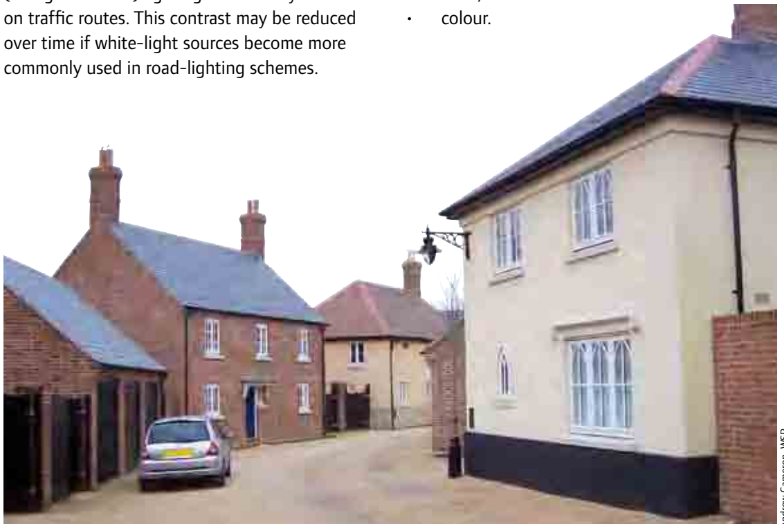
Figure 10.3 Street light mounted on a building.
