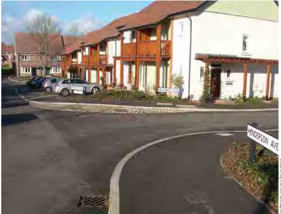
Figure 7.25 The overrun area at this junction is hazardous for pedestrians and/or requires them to divert from their desire line. Notice also the unsightly placing of inspection covers. The layout is particularly hazardous for blind and partially-sighted pedestrians.
