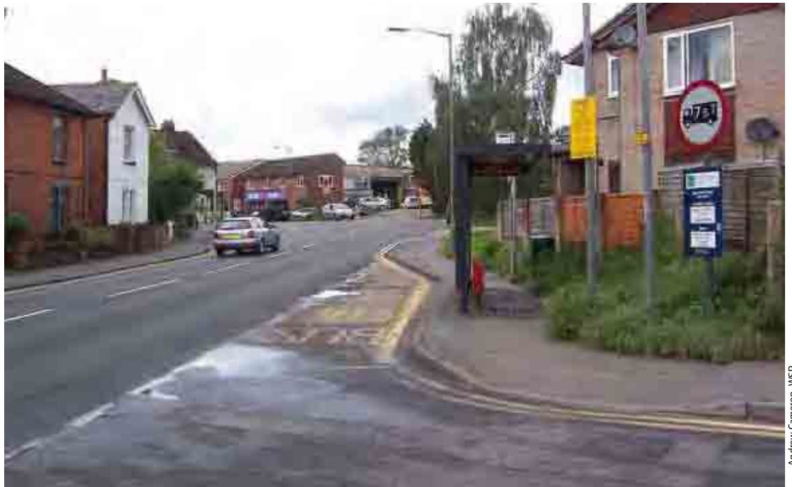
Figure 6.17 The bus lay-by facilitates the free movement of other vehicles, but it is inconvenient for pedestrians.
