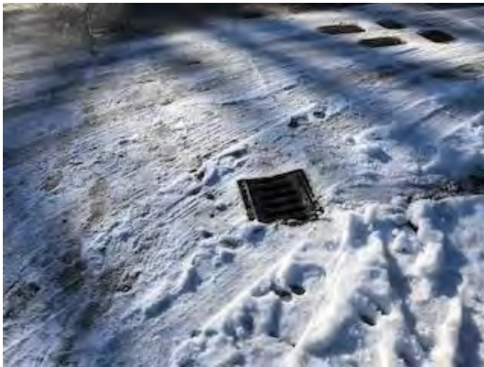
Figure 2: Existing gullies at proposed crossing.
