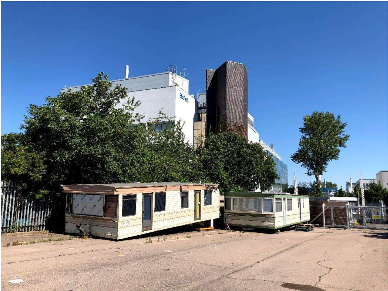
Figure 44. View of the main buildings within the site from within the area of hardstanding to the south.
