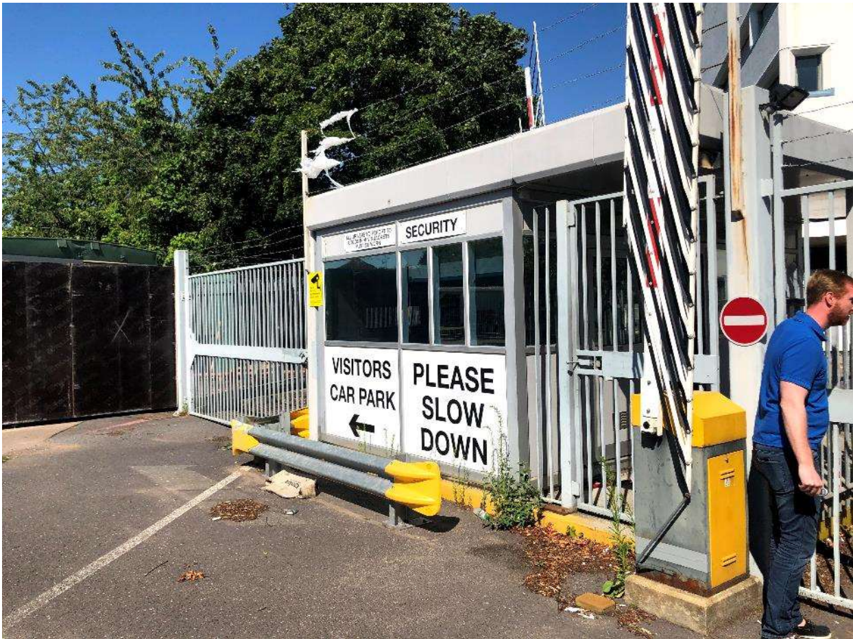
Figure 23. Prefabricated buildings within the site surroundings.
