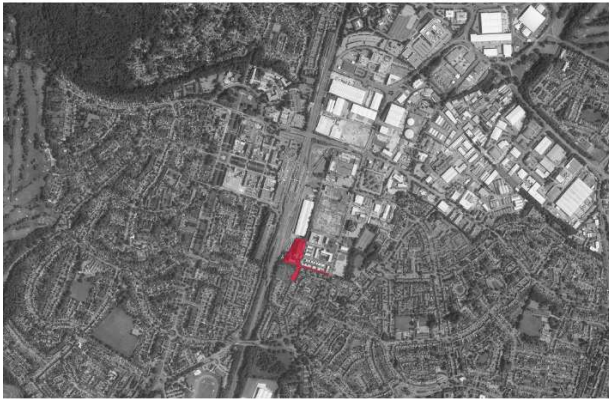
^ Site Aerial View
