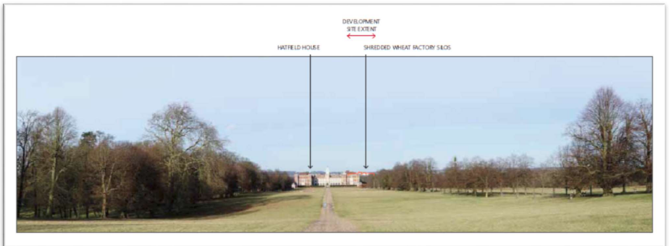
Figure 67. View towards the site from the south of Hatfield House. Please note the buildings within the site are obscured by Hatfield House however the Shredded Wheat Factory is just apparent. The extent of the consented development surrounding the Shredded Wheat Factory is marked in red. Please note this view is reproduced from consented application 6/2018/0171/MAJ.
