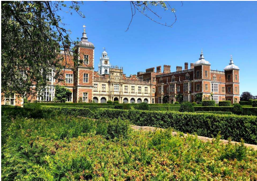
Figure 56. Old south front of Hatfield House, Grade I.
