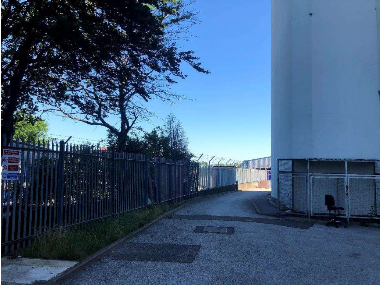
Figure 31. View north looking along the railway line to the sheds to the north.
