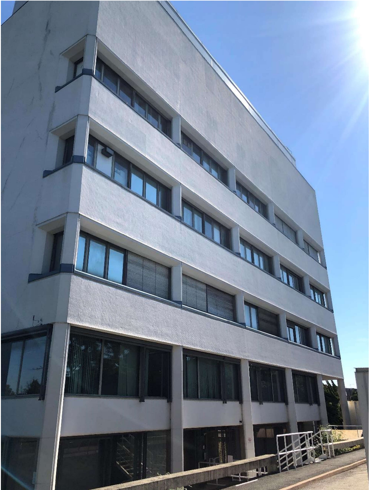
Figure 35. Side elevation, the building is of indifferent design.
