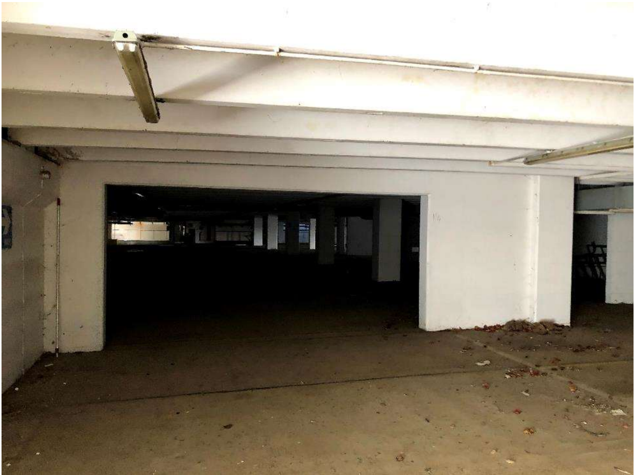
Figure 43. Underground carpark underneath the site.
