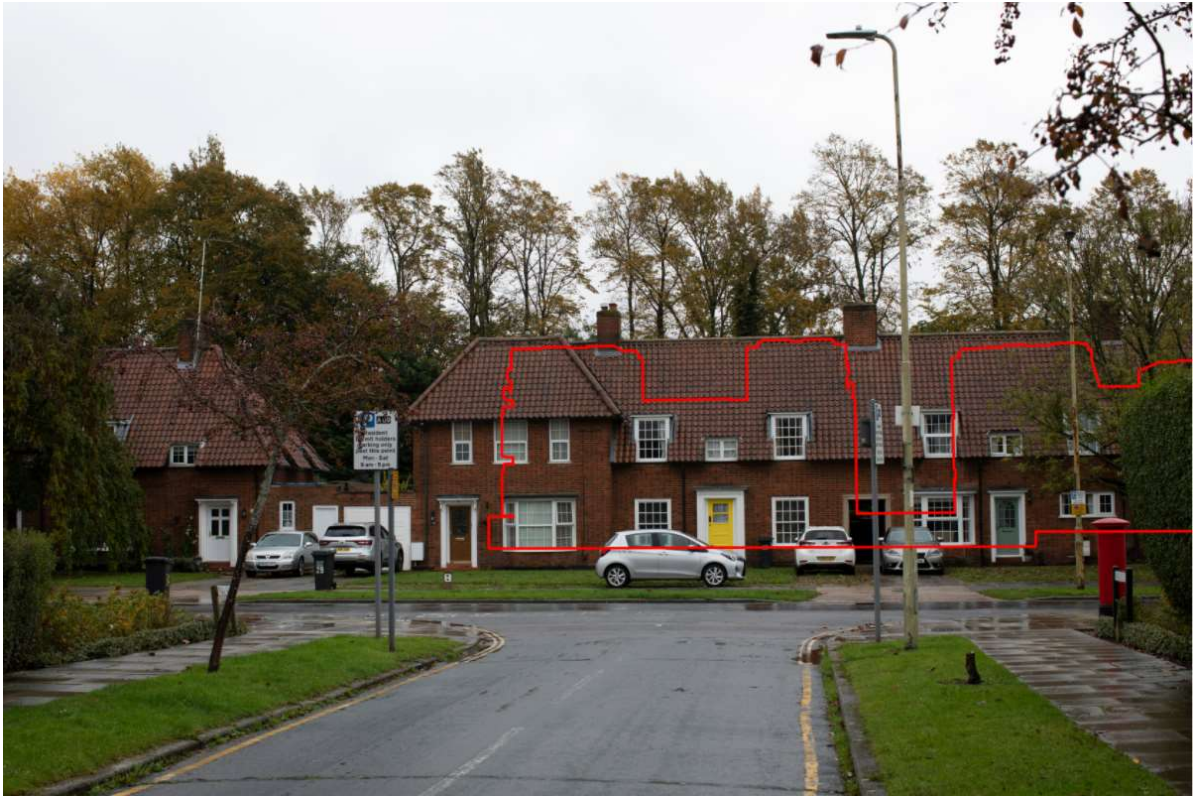
Figure 101. Verified View 1. Summer View. Red line indicates the outline of the proposals.
