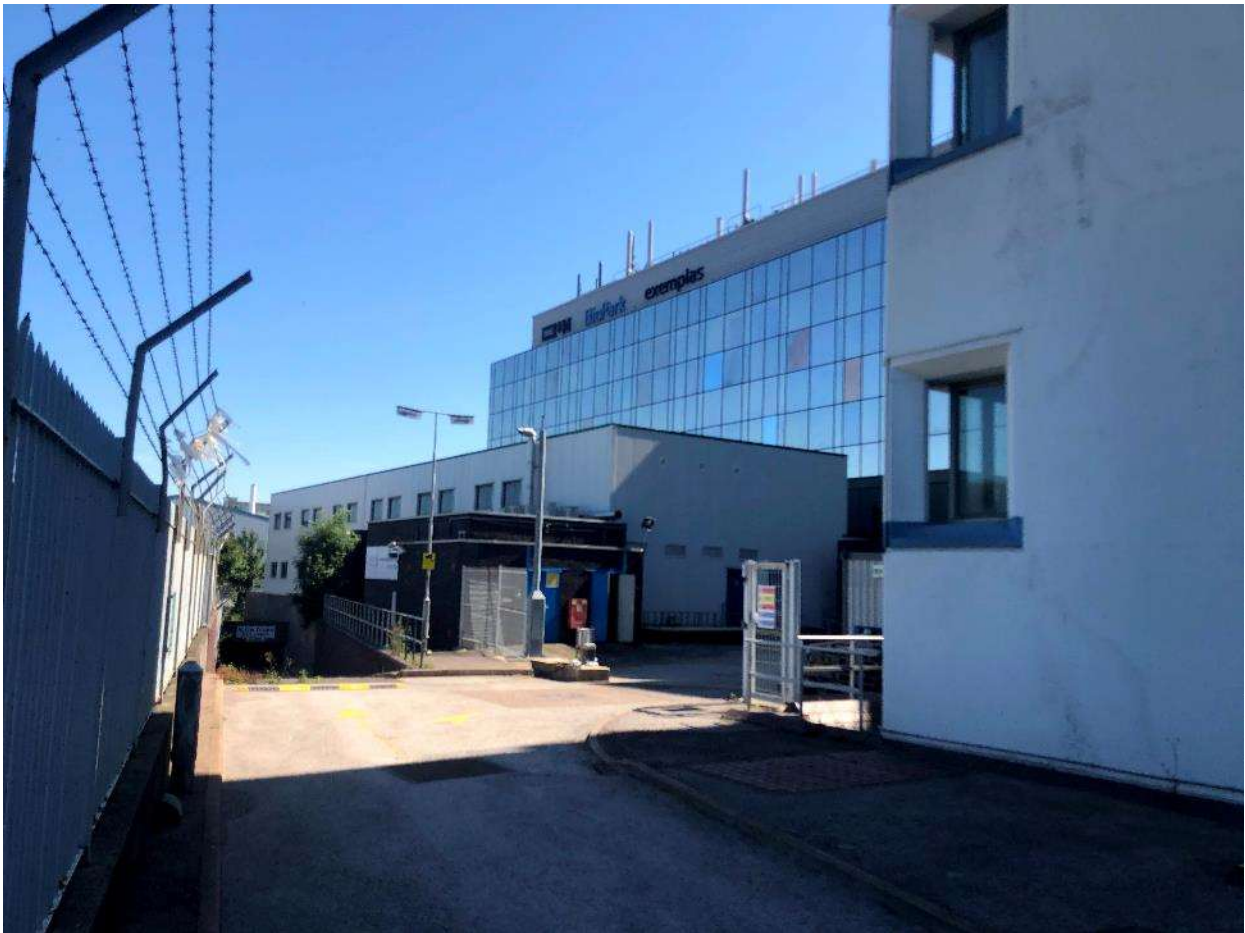
Figure 34. Side elevation of the Biopark building, note the utilitarian design.
