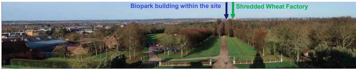
Figure 60. View from the roof of Hatfield House looking towards the site. Note the red line indicating extent of consented redevelopment surrounding the Shredded Wheat Factory. To the left of the image the development along the Great North Road can be seen, as can the surroundings of Hatfield. Please note this view is reproduced from consented application 6/2018/0171/MAJ due to limited access to the house and garden.
