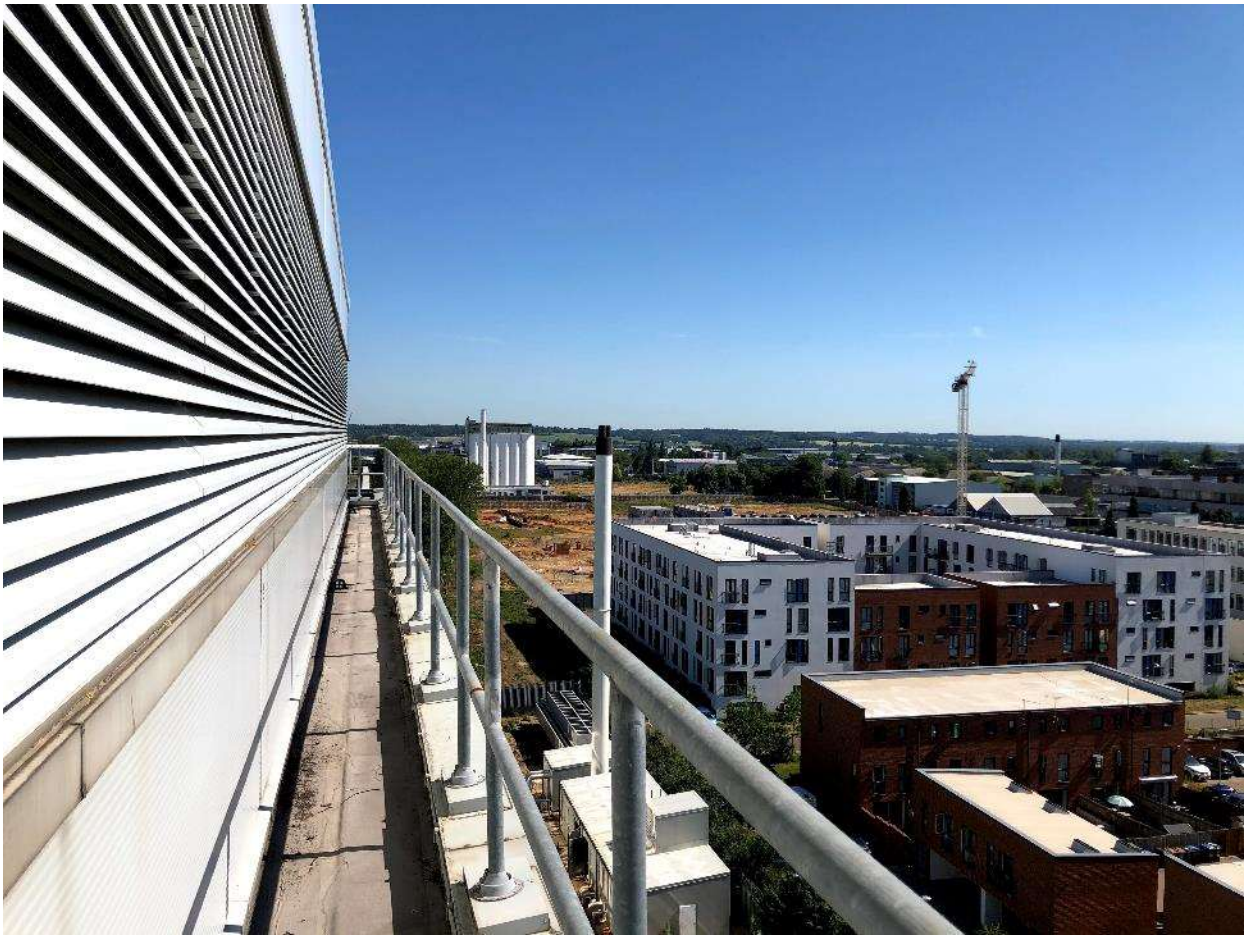
Figure 38. View north towards the Shredded Wheat Factory.
