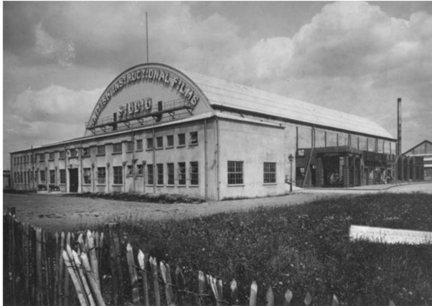
Figure 10- Welwyn Studios now demolished
