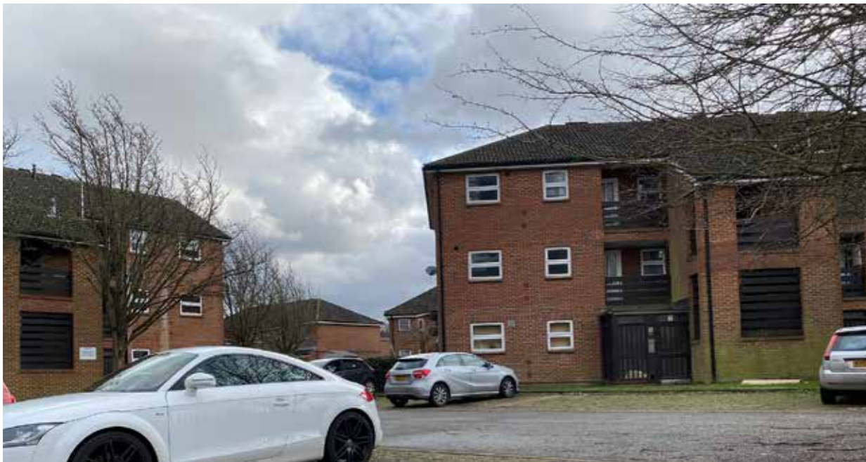
^ Three storey flats Broadwater Crescent
