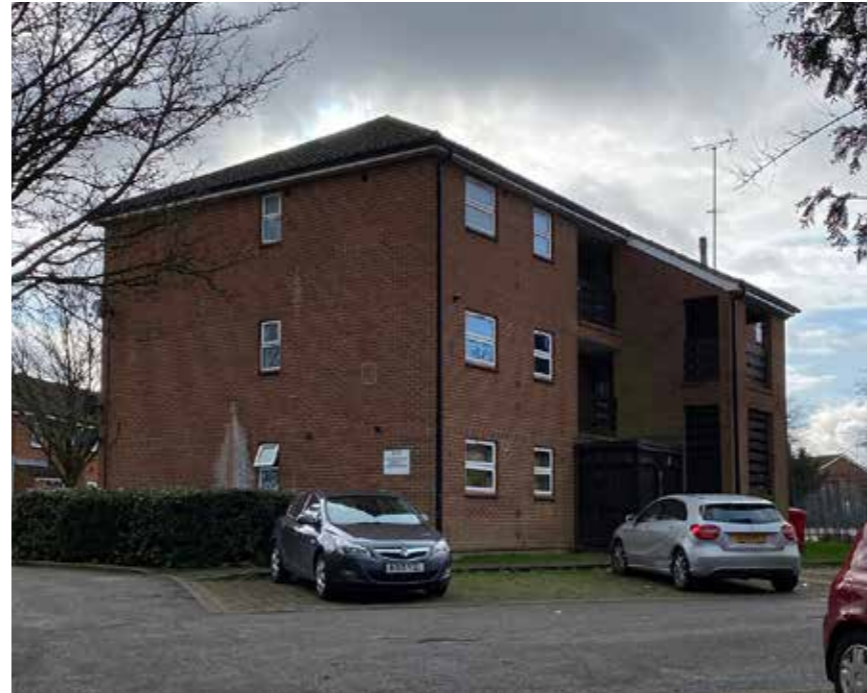
^ Three storey flats Broadwater Crescent
