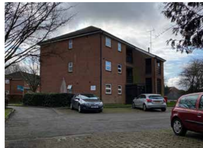
5. Broadwater Crescent and vicinity: Red brick residential buildings with pitched roofs
