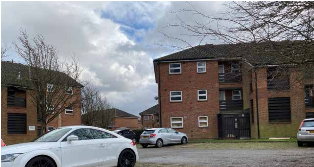
^ Three storey flats Broadwater Crescent
