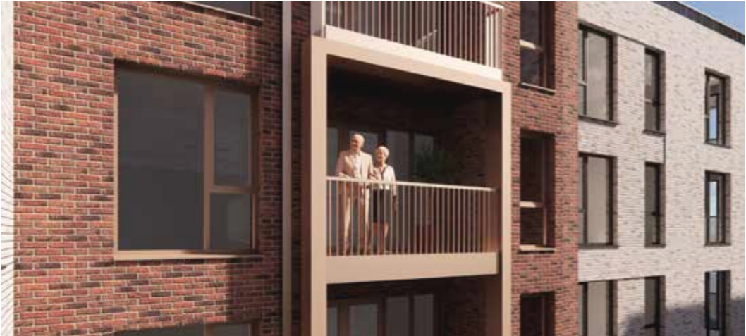
^ Bronze frames surrounding inset balconies within red brick
