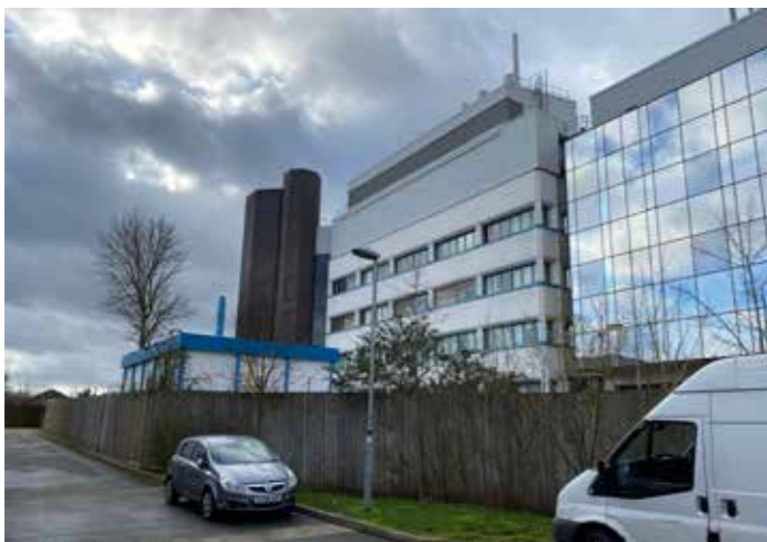
SITE: BioPark laboratories: White render, glass, metal, masonry industrial building (refer to section 2.1 for further details)
