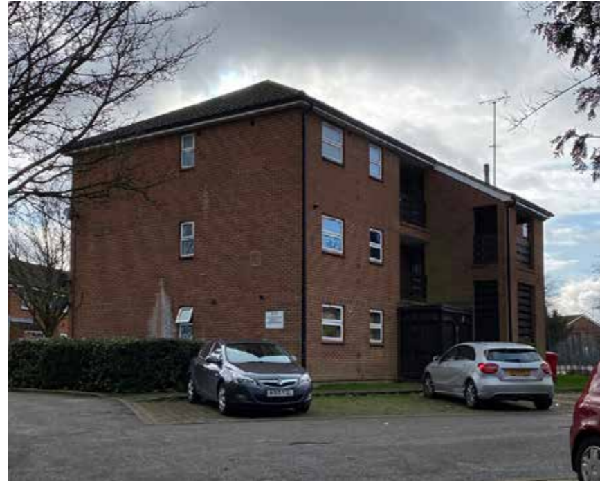
^ Three storey flats Broadwater Crescent
