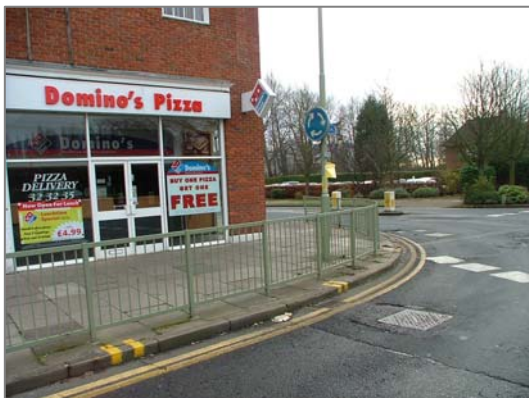
Discordant 1970's architecture, poor shopfronts guardrail and painted lines mar original style.
