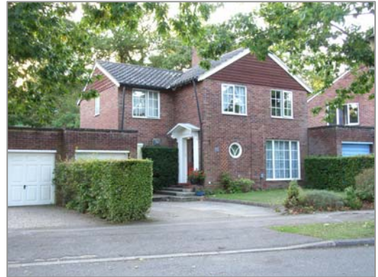
Templewood has sensitive scale and detailing, but uPVC window replacements undermine authenticity.
