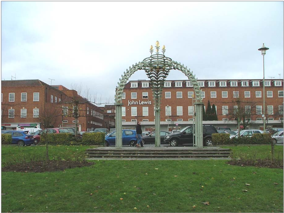
The Anniversaries Garden functions as a public space and provides a pedestrian link between Stonehills and John Lewis.
