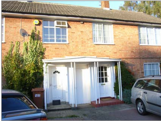
1950's houses adjoining Knightsfield with original detailing
