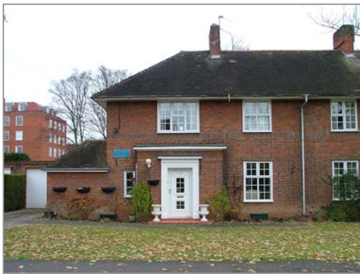
Despite UPVC door and window replacements, 5 Guessens Road, the former home of Ebenezer Howard, is recommended for statutory listing.
