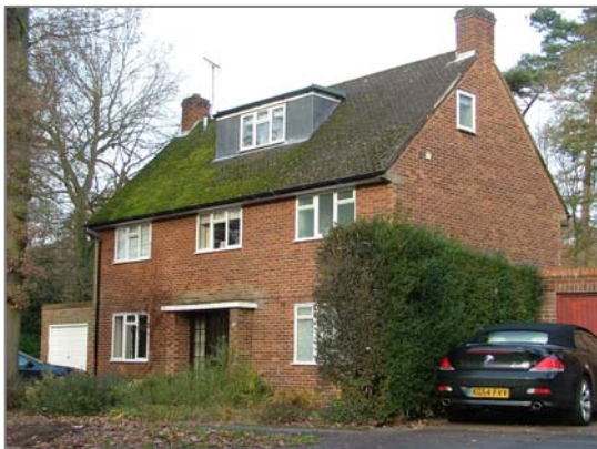
Later, post de Soissons approach at The Reddings, with houses set in leafy surroundings.
