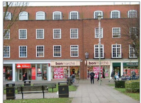
Well scaled detailing above shopfront level in Howrdsgate is compromised by overly dominant facias.
