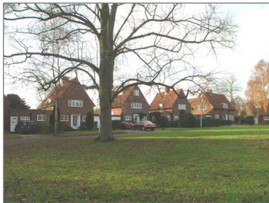
Houses in Barley Croft Green have been extended with single storey garages. Rhythm, form and views have been maintained, preserving overall character.
