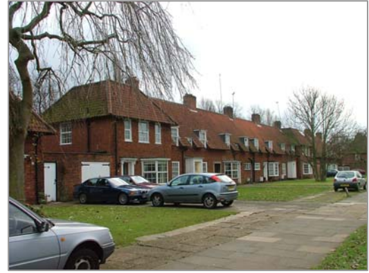
Longcroft Lane streetscape: Projecting end properties add visual interest to the uniformity of the group.
