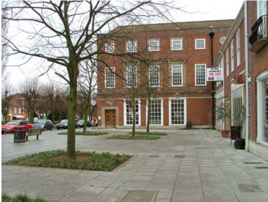
The HSBC building and former estate department of Welwyn Garden City Ltd - an example of de Soissons's civic neo-Georgian
