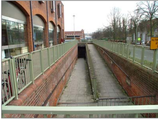
Subway and guardrails at Church Road
