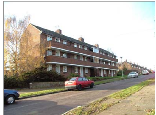
Balcony access flats at Stanborough Green
