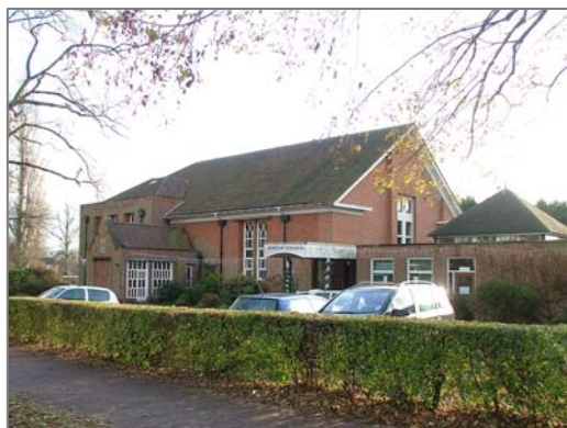
Red brick simplicity extends to the Garden City's ecclesiastical architecture, as the Church of St Francis of Assisi shows.
