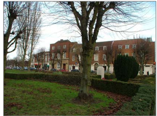
View across Howardsgate towards the former Barclays Bank (now ‘The Cork’)
