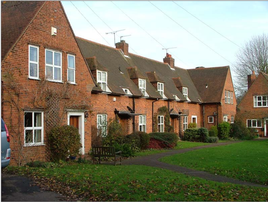
An Arts and Crafts language defines the architecture of The Orchard. Note however the inappropriate replacement glazing materials that can erode the group's integrity.
