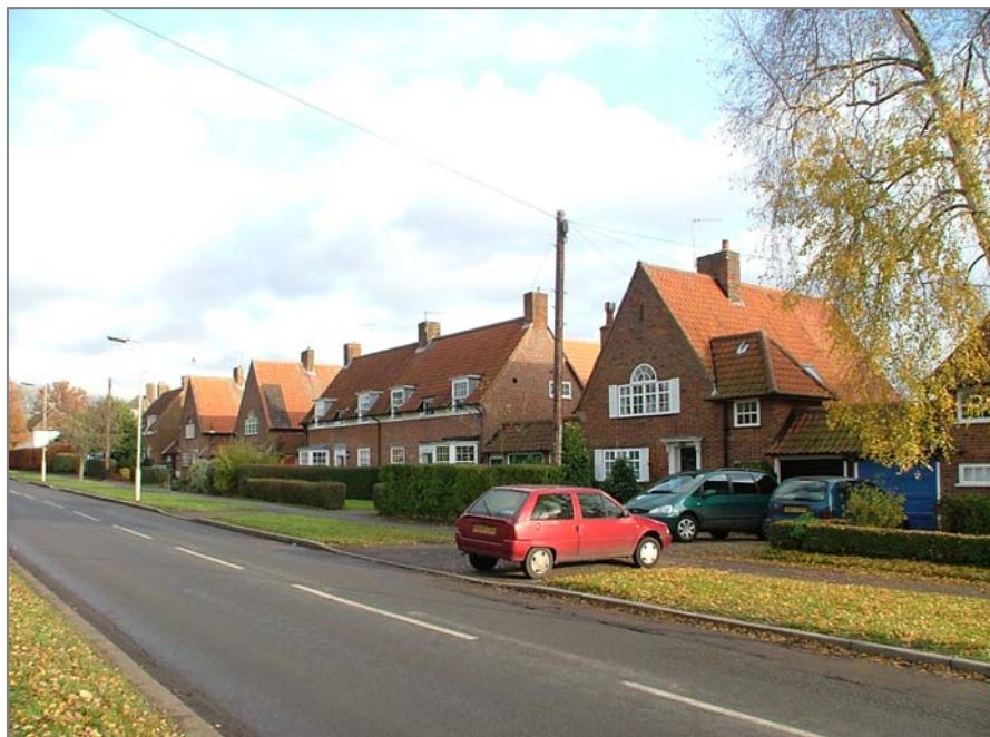
Steeply roofed gabled houses in The Old Drive. Garage extensions are later additions.
