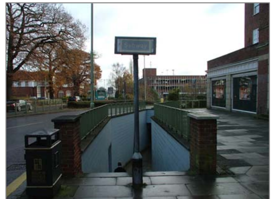
Subway at Bridge Road testifies to difficult pedestrian circulation in this area.
