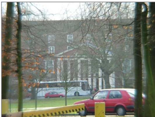
The former Welwyn Stores (now John Lewis)
