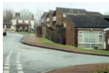
1970's split gable and monopitch houses, typical of the period. Note the tighter layout.
