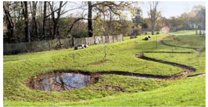
Attenuation ponds retain run-off and remove contaminants before draining into a water course.
