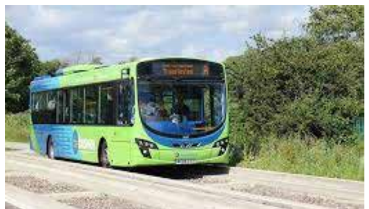
The Cambridge Busway is an examples of a solid sub-structure road that can read as a 'lane'.
