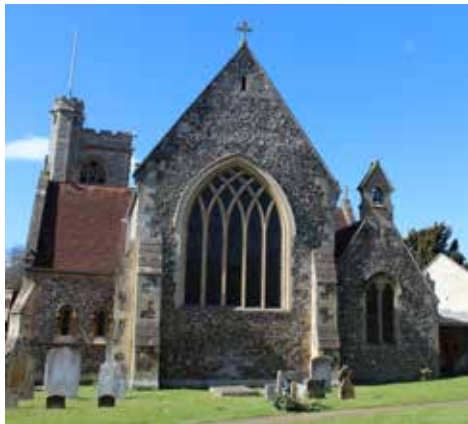
Figure 31 Church of St Mary, eastern elevation
